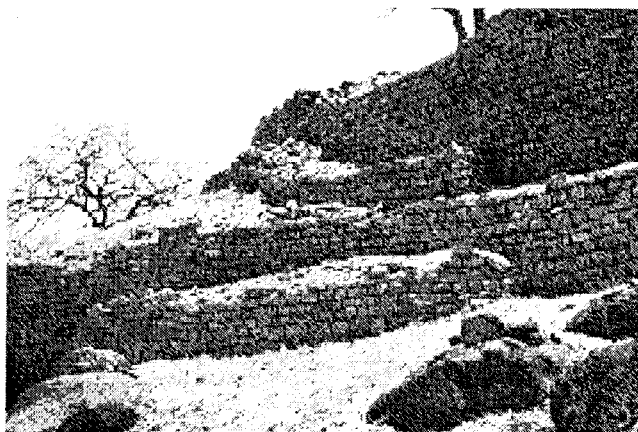
Fig. 9. Retaining dry stone walls at Khami, Zimbabwe.
