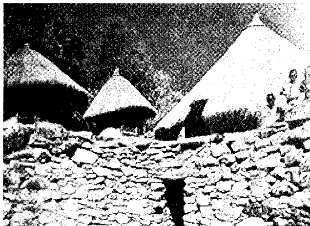
Fig. 8. Undressed stone “kraal” with daga as cement and daga huts above in Manyika Eastern Highlands, Zimbabwe.
